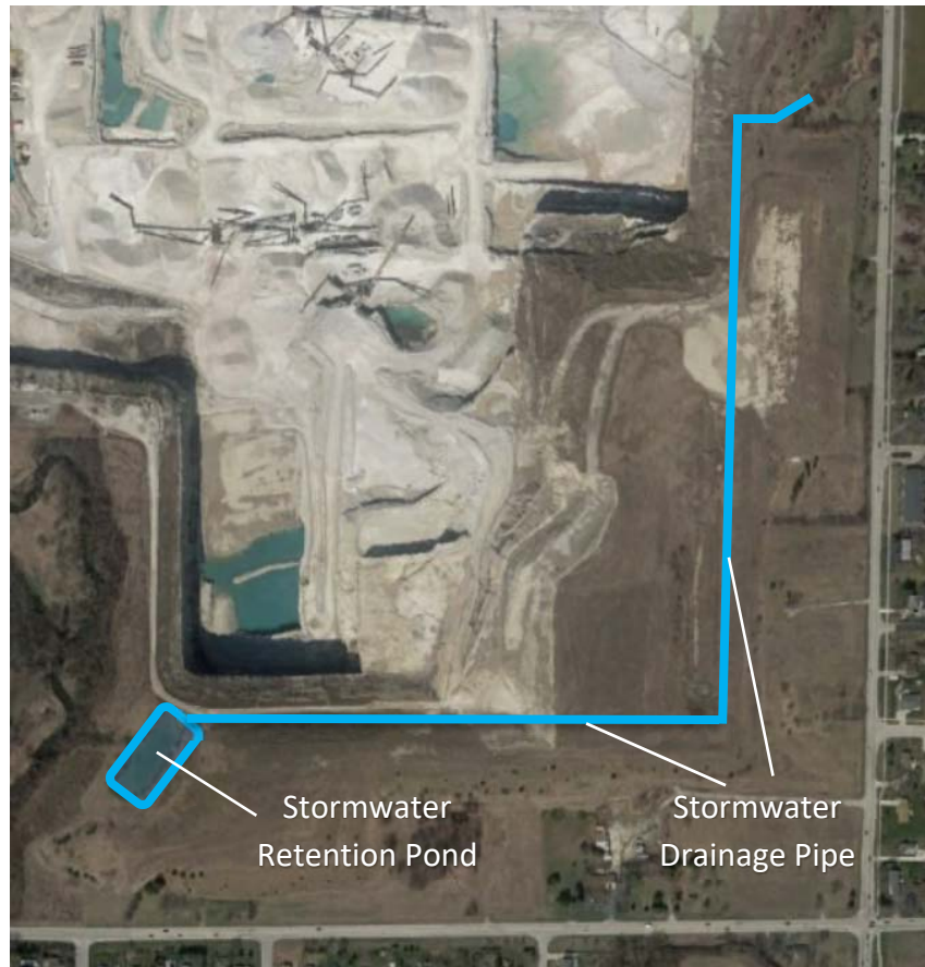
Photo Showing Approximate Location of Stormwater Drainage Pipe and Retention Pond
