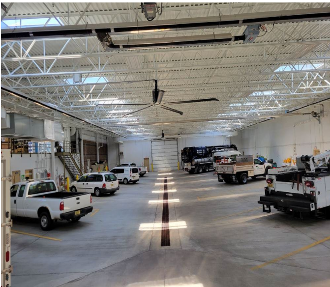
Water Utility Building
