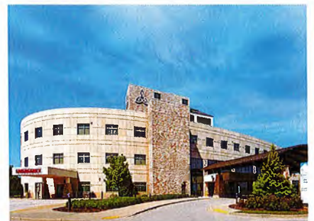
Ascension Hospital - Franklin
