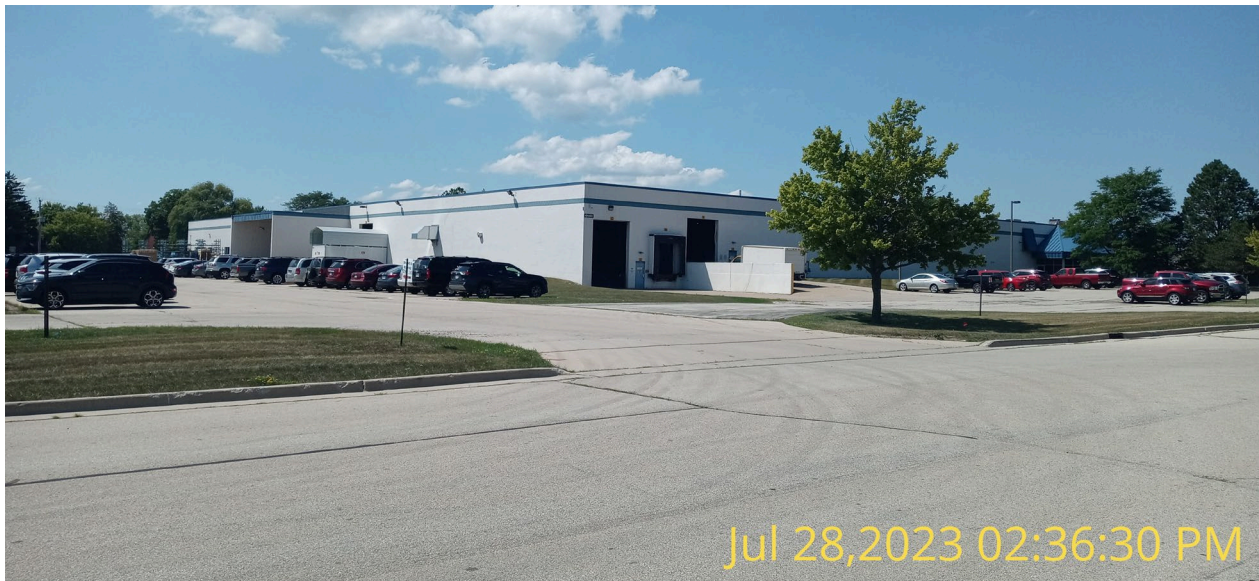
View of the exiting Allis Roller building, note that curb and gutter is installed on S. 57 th Street Photo by City Development staff
