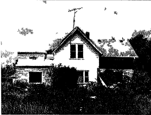
Photo 1) House, Looking at South Side ~2,200 ft 2
