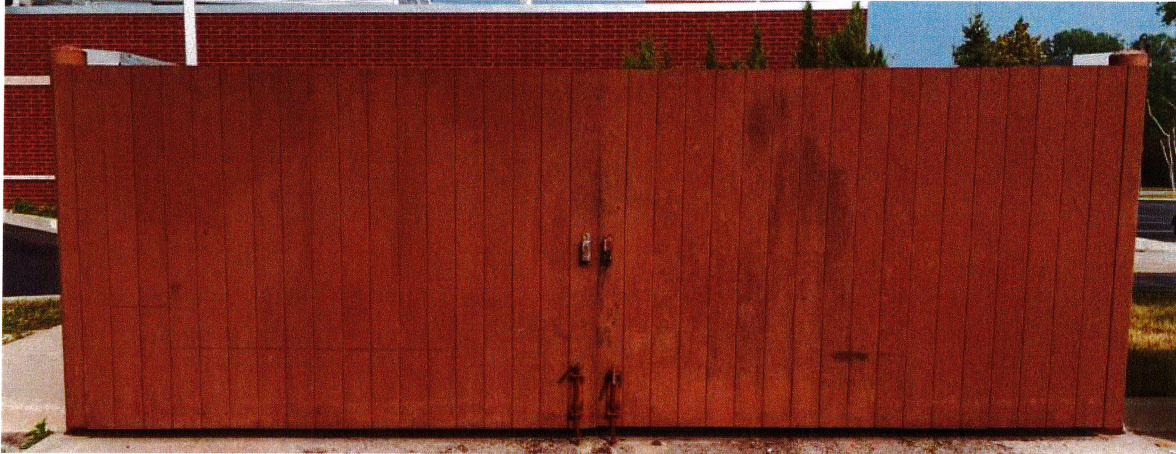
Existing trash enclosure fencing / gate (Proposed fence enclosure to be similar)
