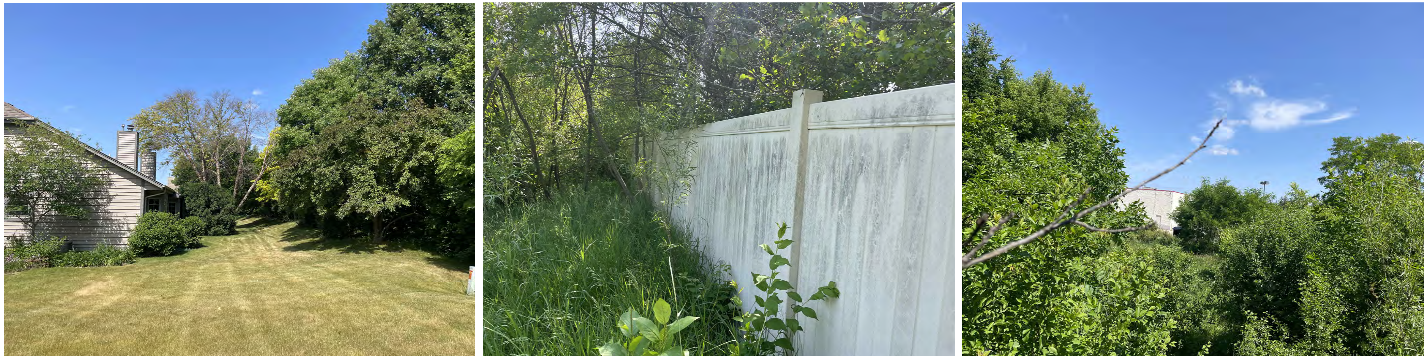
B EXISTING CONDITION PHOTOS
