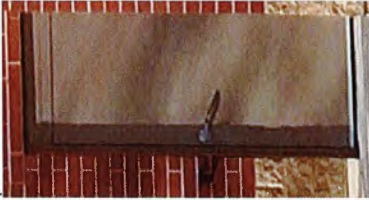
PAINTED HOLLOW METAL SERVICE DOOR AND FRAME (COLOR TO MATCH ADJACENT MASONRY).
