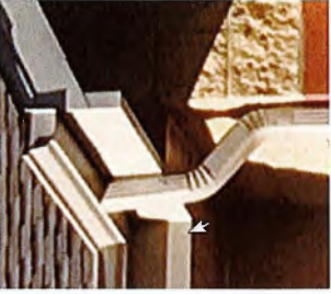
PREFINISHED METAL DOWNSPOUT AND GUTTER SYSTEM
