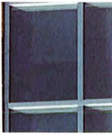
CLEAR ANODIZED STOREFRONT WINDOW WITH THERMALLY BROKEN CLEAR ANODIZED FRAME AND 1" CLEAR AGC LOW E #3 GLASS (TEMPERED WHERE REQUIRED PER CODE)
