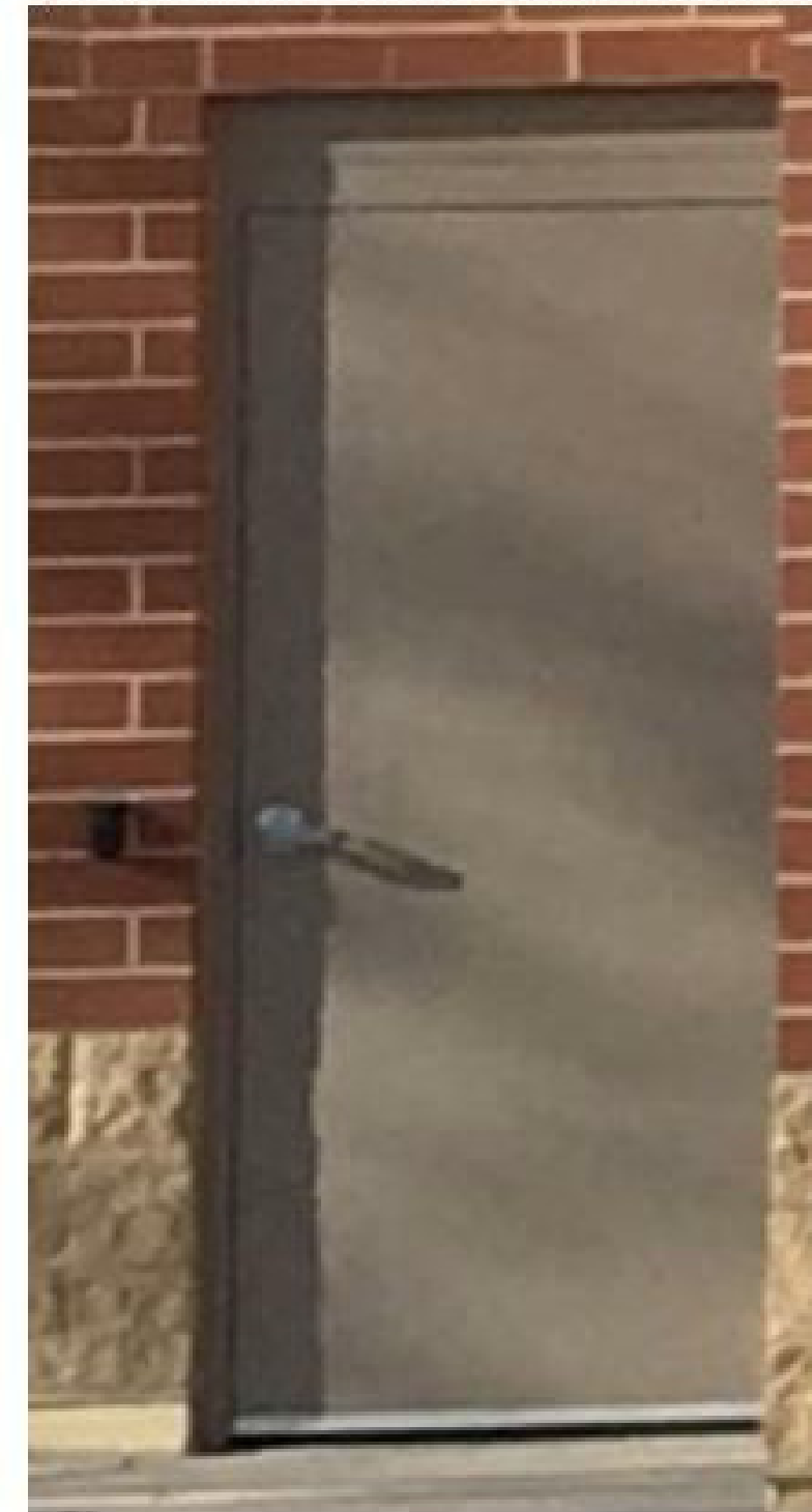
PAINTED HOLLOW METAL SERVICE DOOR AND FRAME (COLOR TO MATCH ADJACENT MASONRY).
