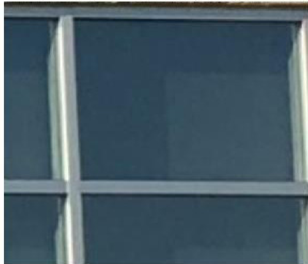
CLEAR ANODIZED STOREFRONT WINDOW WITH THERMALLY BROKEN CLEAR ANODIZED FRAME AND 1" CLEAR AGC LOW E #3 GLASS (TEMPERED WHERE REQUIRED PER CODE)
