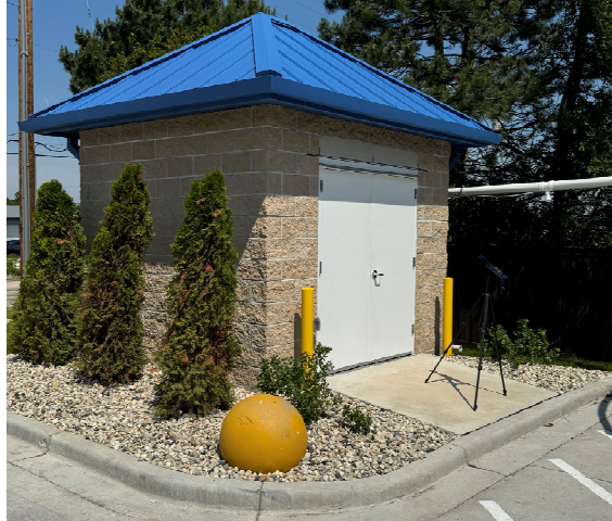
Figure 6: Vacuum Pump House
