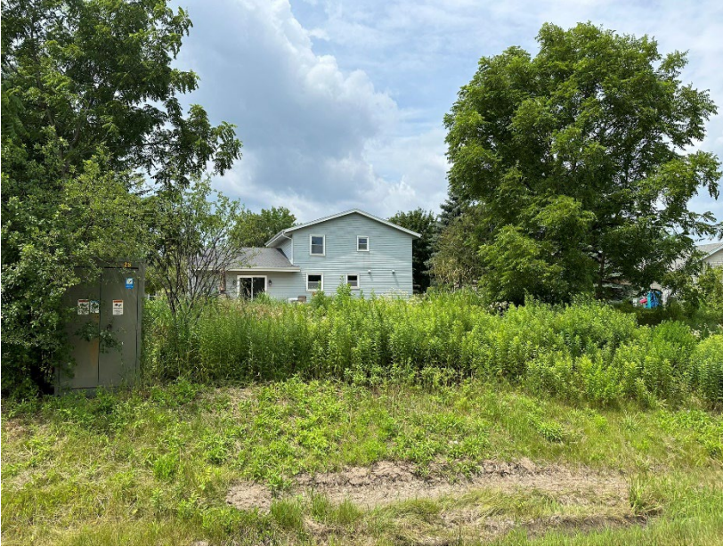
View of the berm on the west side of 76 th Street, from roadside looking west.
