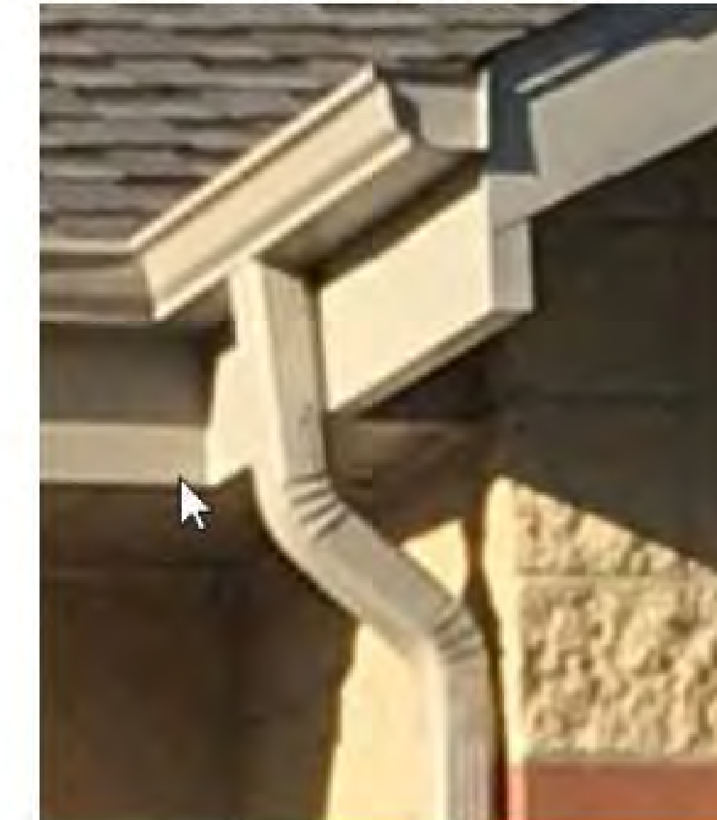
PREFINISHED METAL DOWNSPOUT AND GUTTER SYSTEM
