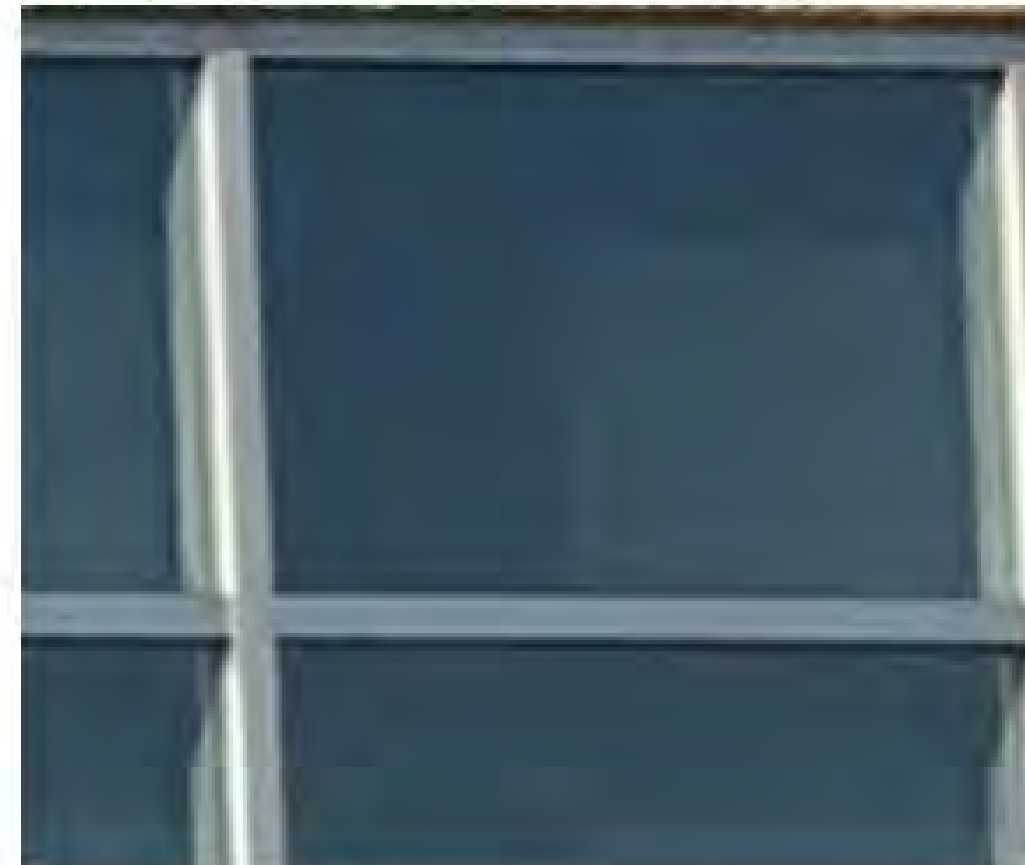
CLEAR ANODIZED STOREFRONT WINDOW WITH THERMALLY BROKEN CLEAR ANODIZED FRAME AND 1" CLEAR AGC LOW E #3 GLASS (TEMPERED WHERE REQUIRED PER CODE)
