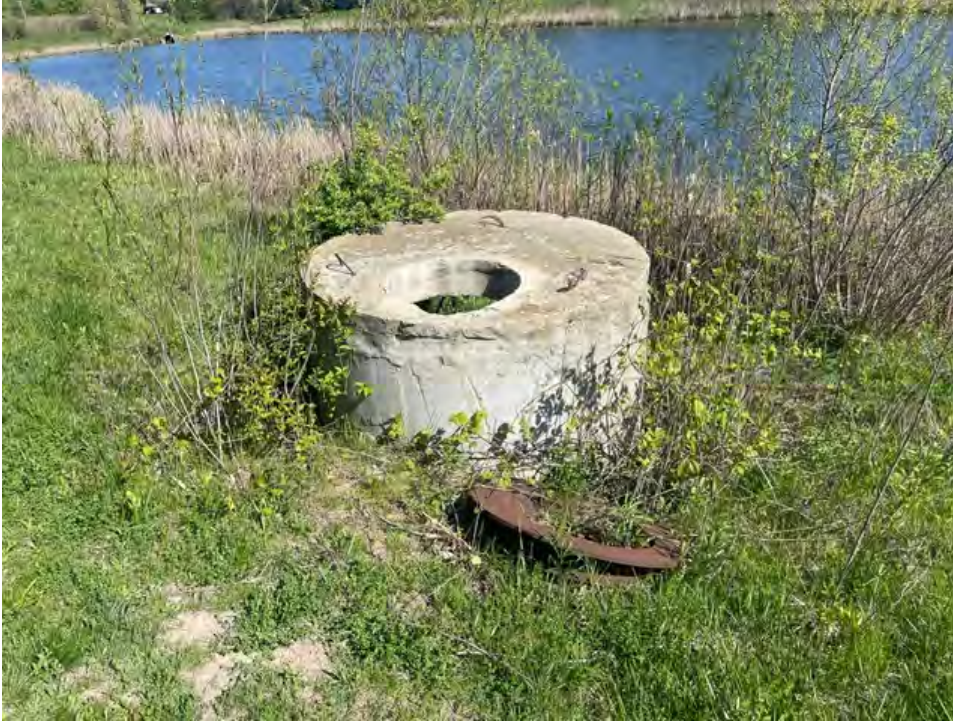
Fig 1: Pond outlet structure (May 6, 2024)
