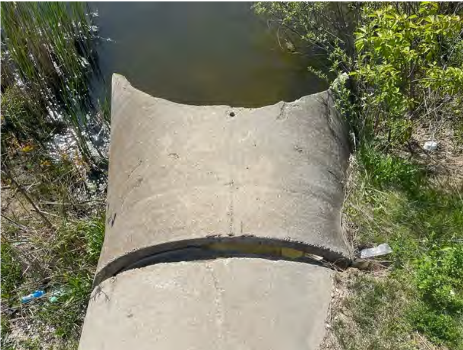
Fig 2: Pond inlet end section located at southeasterly corner of pond (May 6, 2024)
