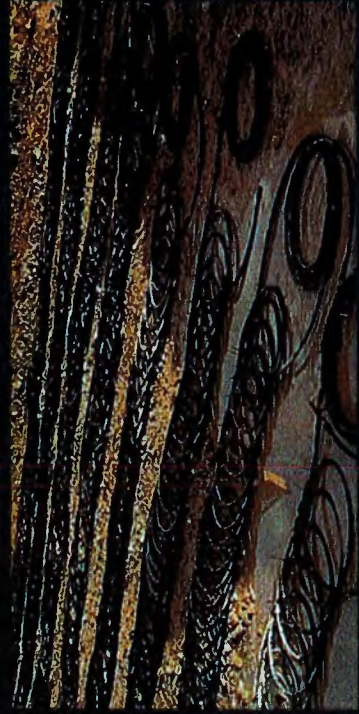
HDPE "Slinky" geothermal coils
