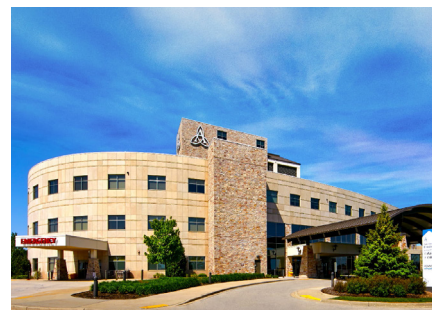
Ascension Hospital - Franklin
